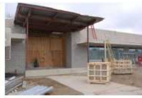
Entry – River Place West
